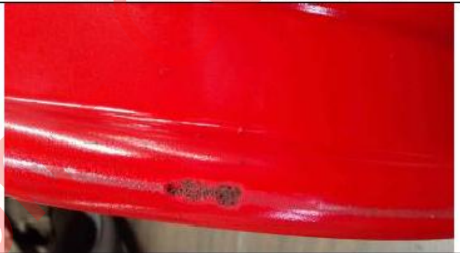
Coating Scuffed off (around 5cm) -Maj
